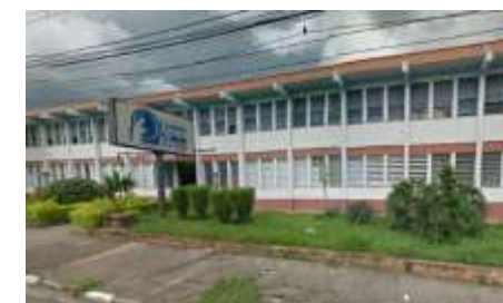
Hospital Álvaro Ribeiro Fonte: Google Street View (2014).
